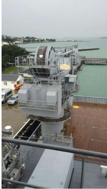
Manawanui - 100 tonne crane
