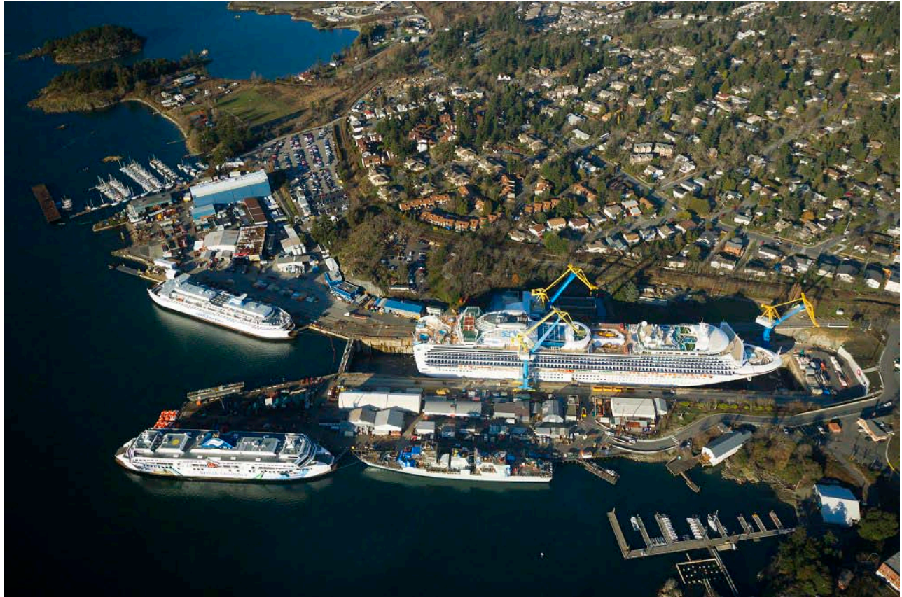
Esquimalt Graving Dock, Victoria, Canada
